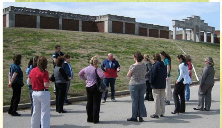
15 SWE members and friends participated in the tour of the Mohawk Water Treatment Plant on March 30th
